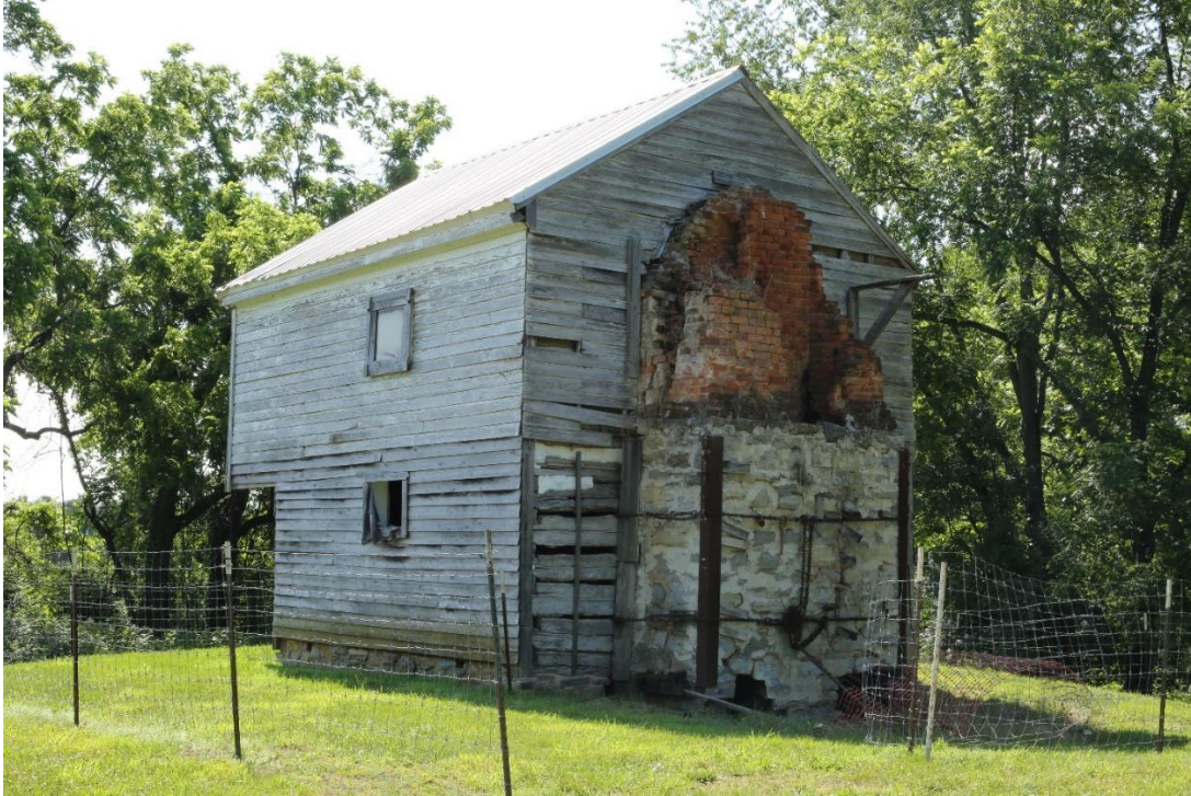
Photo 17: Greenfield Kitchen (VDHR ID 011-5700 / NR No SG100007570), facing southeast.
