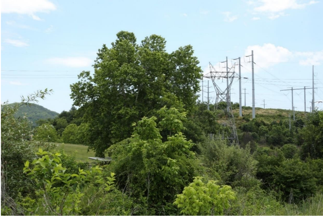
Photo 14: Norfolk and Western Railway Section (011-5481) at bottom foreground obscured by vegetation, from the end of Olde Route 604, facing southeast. Note additional existing transmission lines in the viewshed that connect to Cloverdale Substation.
