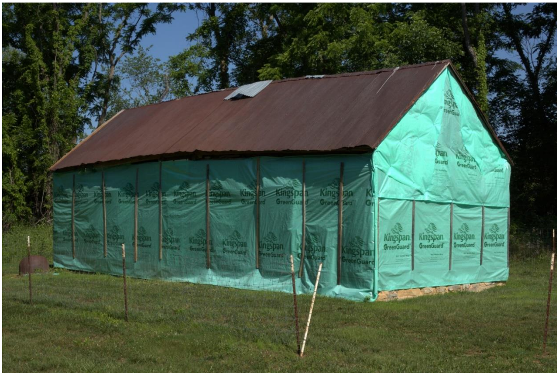
Photo 18: Greenfield Quarters (VDHR ID 011-5700 / NR No SG100007570), facing north.
