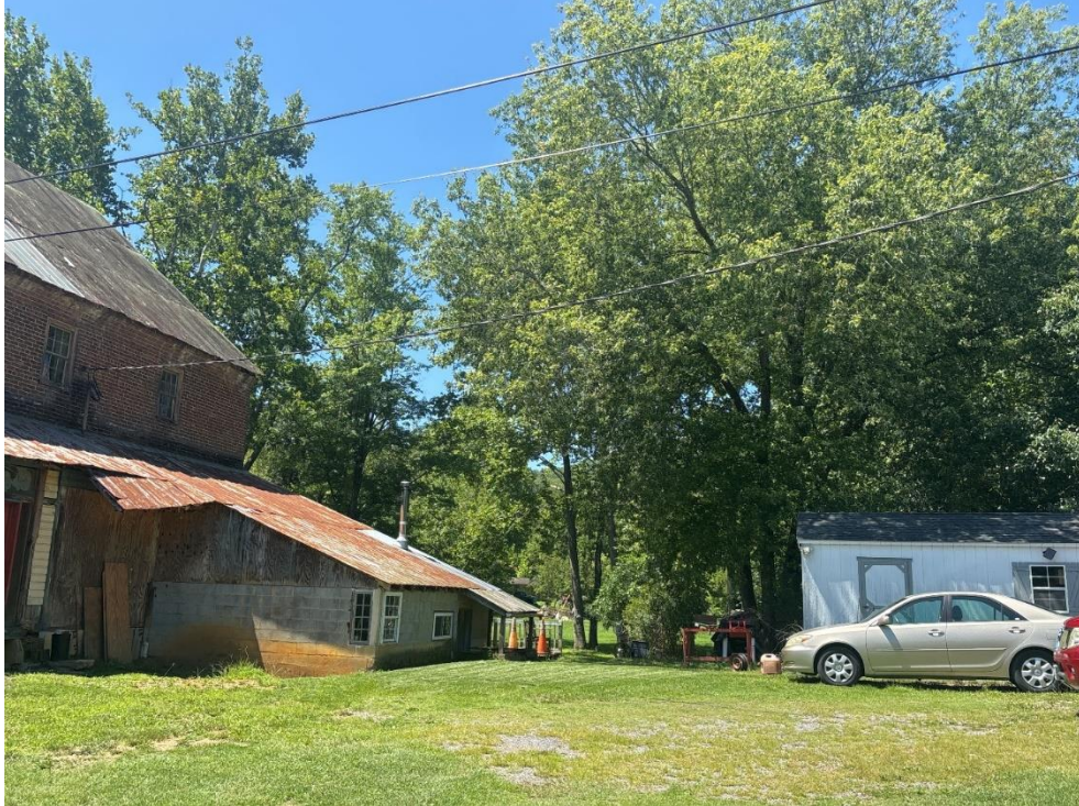
Photo 10: Nininger's Mill-Tinker Mill (011-0057) from Tinker Mill Road with Project in distance obscured by vegetation and topography, facing west.
