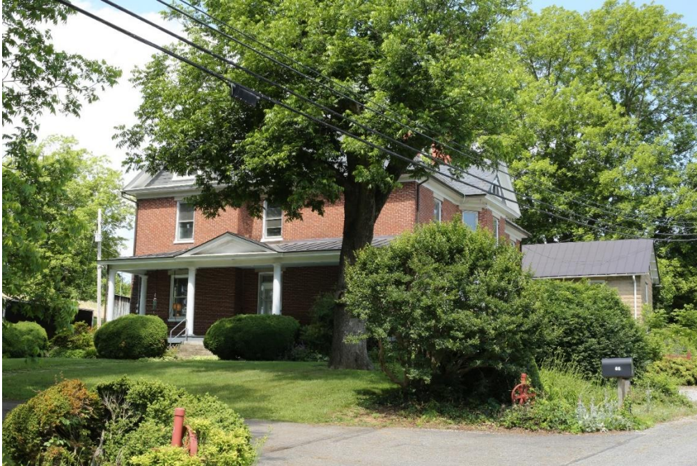
Photo 13: Thomas D. Kinzie House (011-5034) from Kinzie Street, facing northwest.
